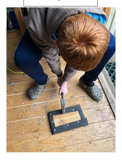
This is the roof. Felt is covering it so it's waterproof. I am using a hammer and nails to keep the felt in the right position.
